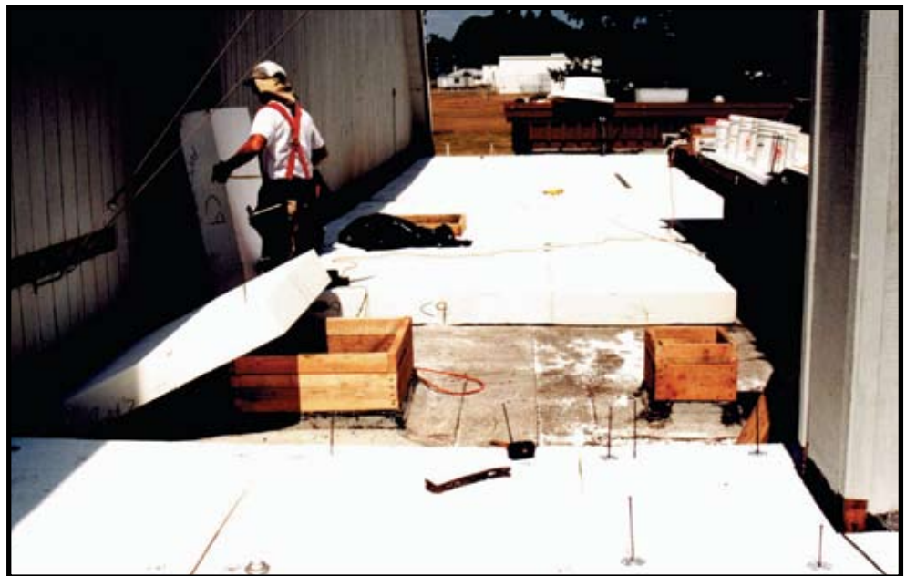
Tapered foam system installed to fill & slope low areas
