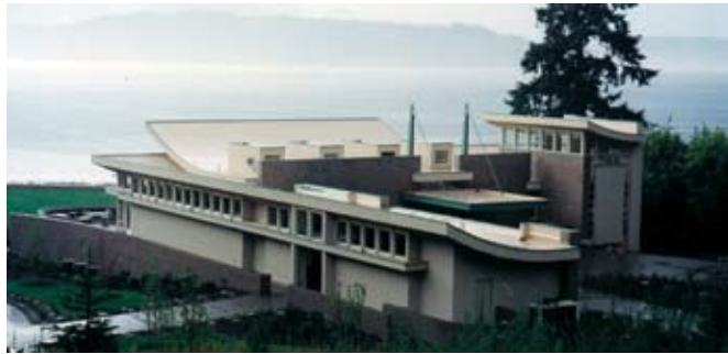
UNIQUE ROOF Requires roofing craftsmanship
